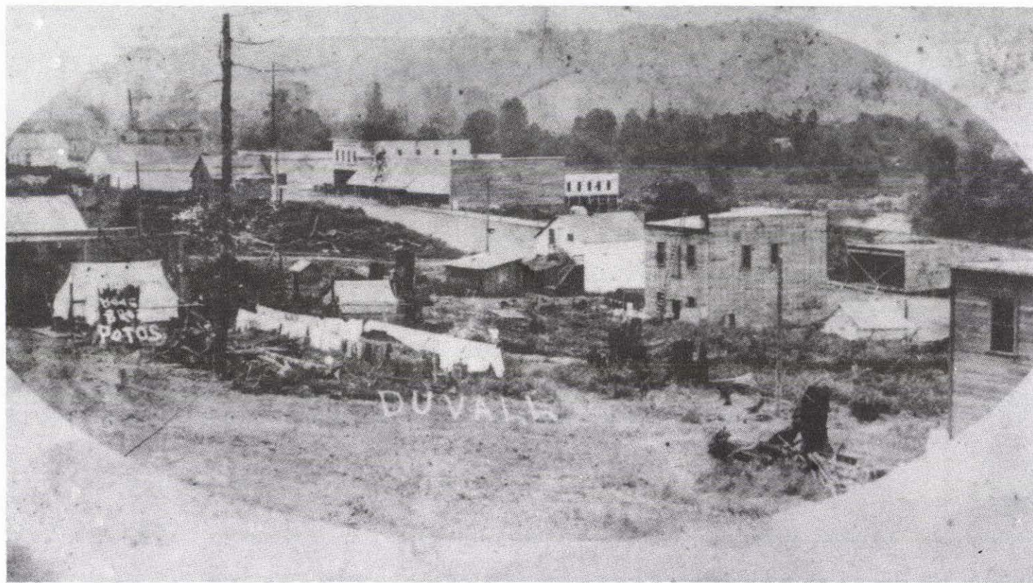
Duvall in 1911, just emerging from its tent city days. The picture was probably taken from Virginia Street. The streets visible are Main and Stewart.
