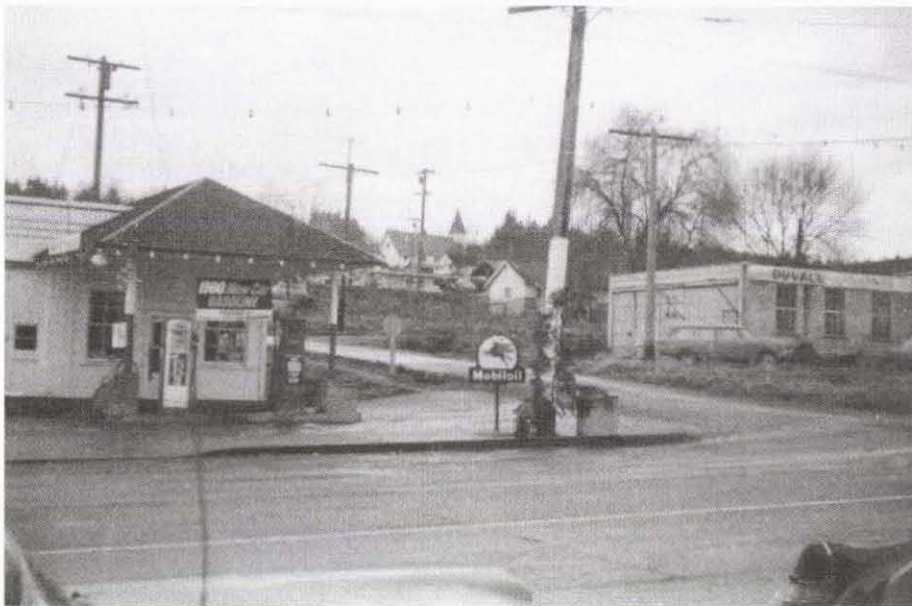
Corner of Main & Virginia Streets – Catholic Church in the background
