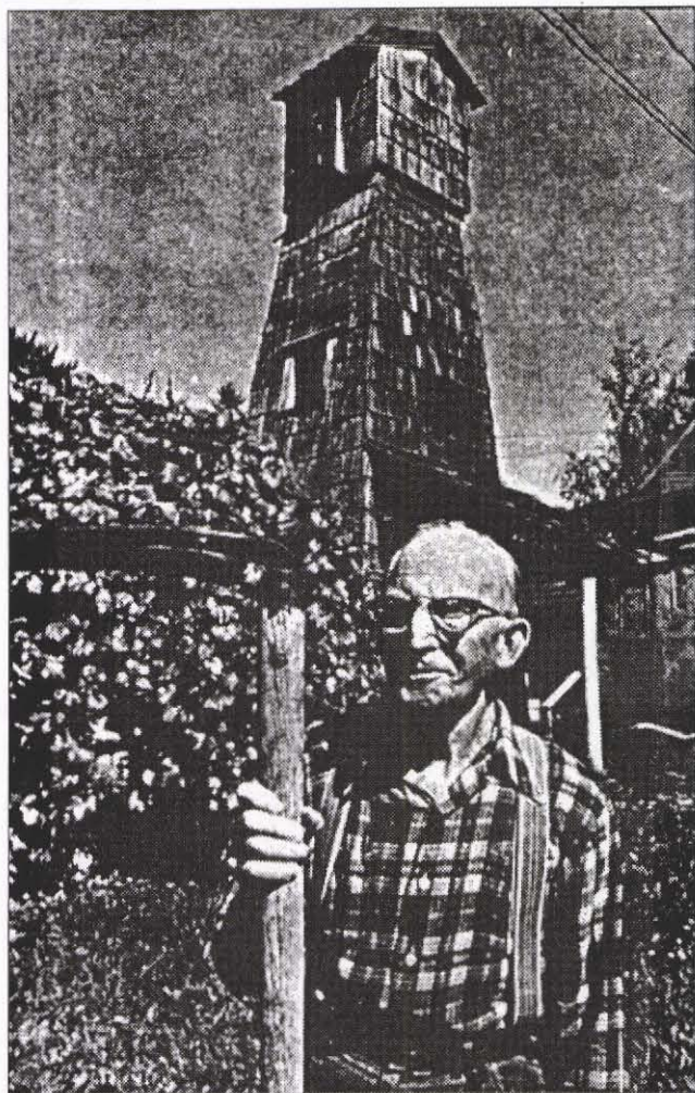
Alva Miller, 85, shown above with the picturesque 3-story tower he constructed in 1936.
