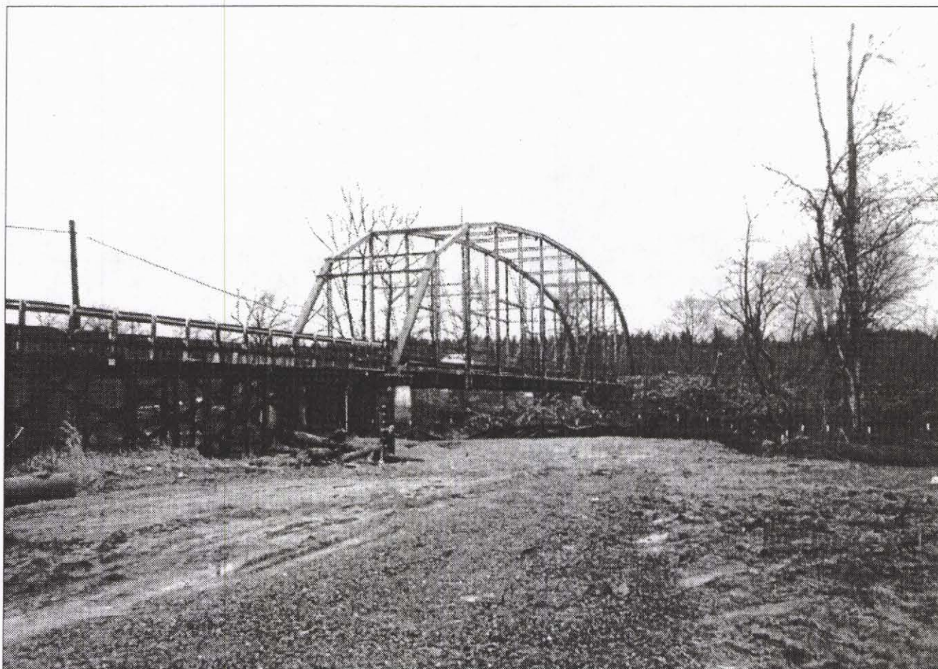
Old bridge at Novelty which was replaced in 2000.
