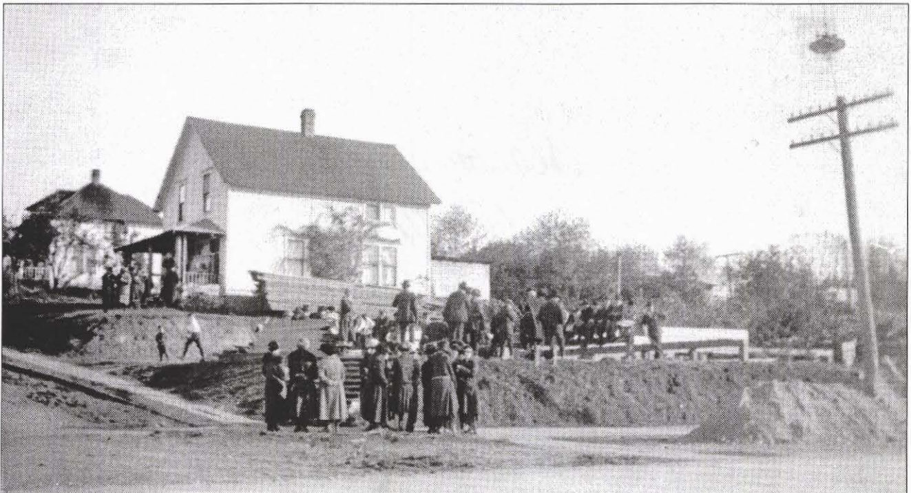
Dr. Roy Pinkerton house – upper house above parsonage. Picture taken 1923 of new church foundation.
